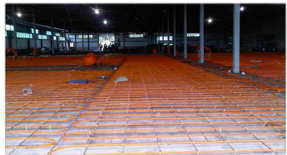
**Over 33 kilometres of hot water piping efficiently heat the bus storage and maintenance areas**
